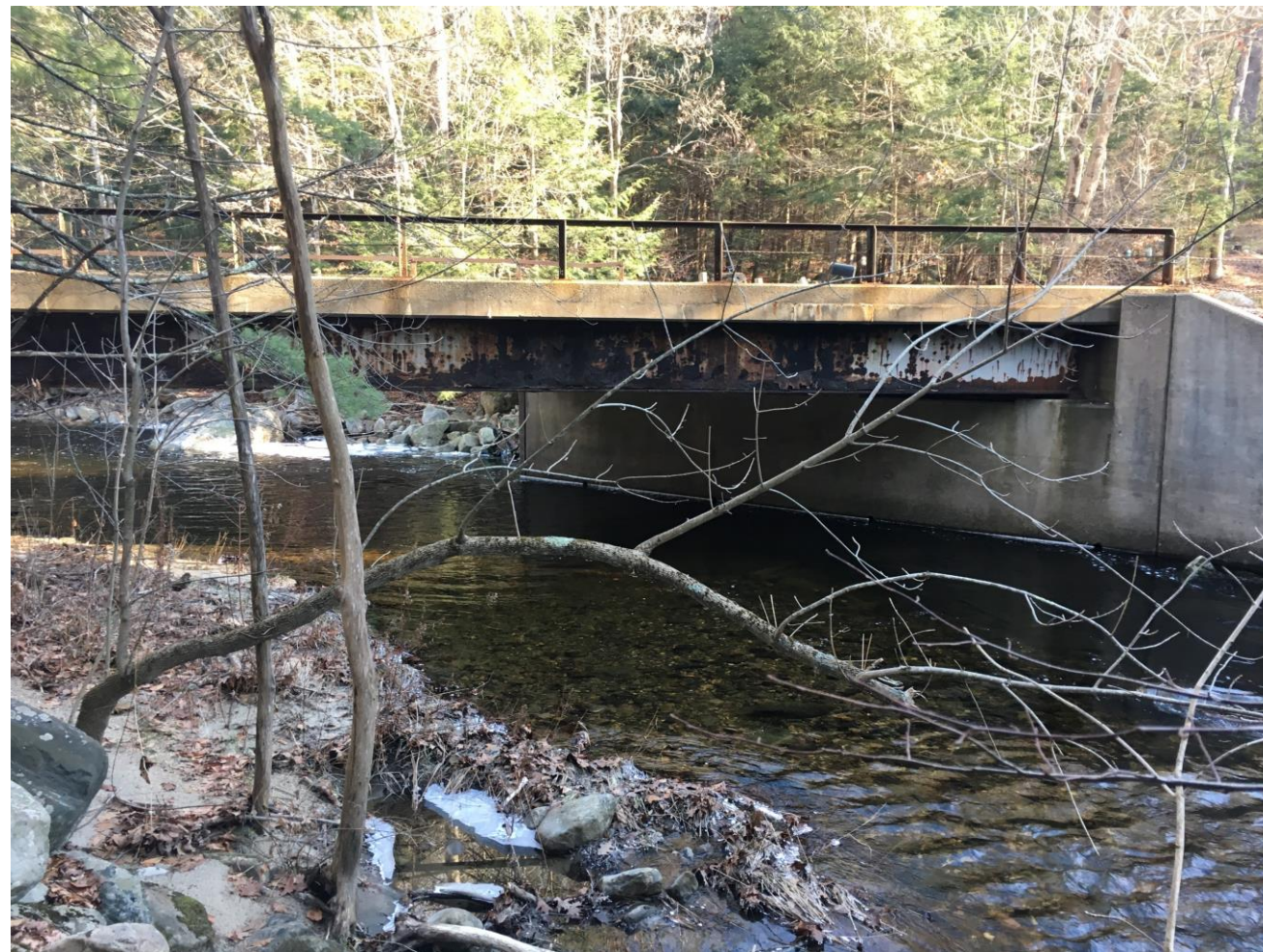
Sandy Brook Road over Sandy Brook
